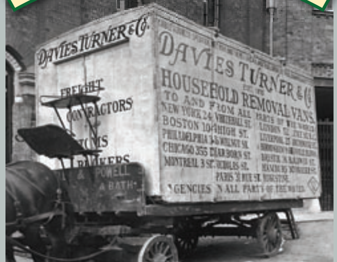
• Davies Turner developed standardised reusable lift-vans like this one, an early precursor to the modern shipping container.
